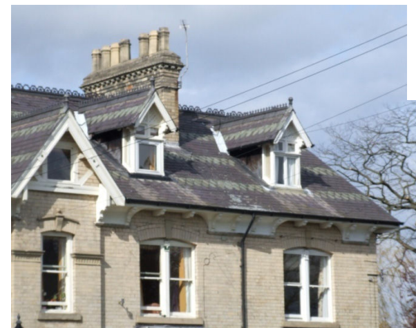
Roof detail Nos 43-45 Heslington Lane
